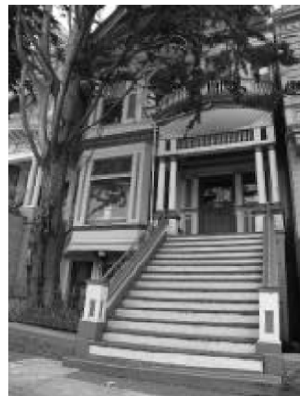
The Department of Building Inspection has looked the other way as two buildings (including 409 Clayton above) leased by the HAFC have accumulated multiple violations.
