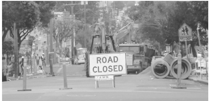
The experimental traffic circle at the intersection of Page and Ashbury has been temporarily removed during sewer replacement work.
