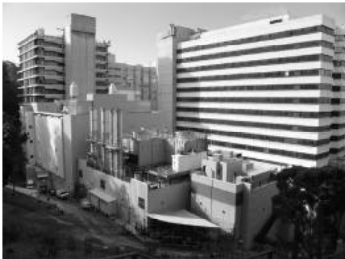
Because of State seismic requirements UCSF will replace three major buildings on its Parnassus campus. (South view above.)
