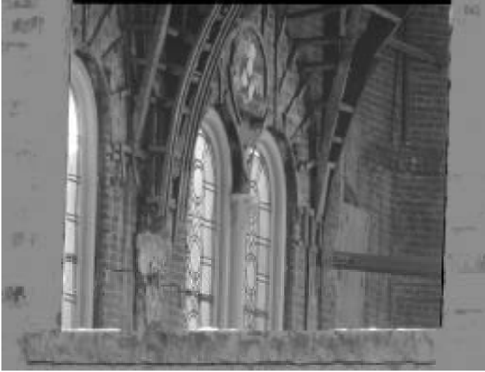
Looing through the rear window, the temporary wooden bracing around the stained glass windows is visible.
